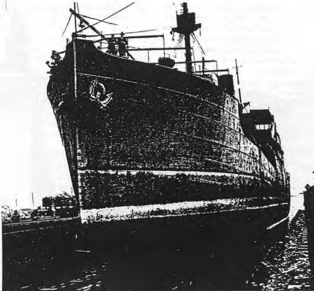
The CHUNGKING high and dry: September 22nd, 1942. With undersides freshly cleaned and antifouled, she went back into the water three days later. (Photocopy courtesy Australian Archives. Accession number MP1587.)
