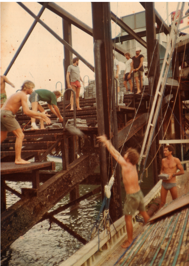
Unloading many tonnes of floor tiles at Darwin wharf
