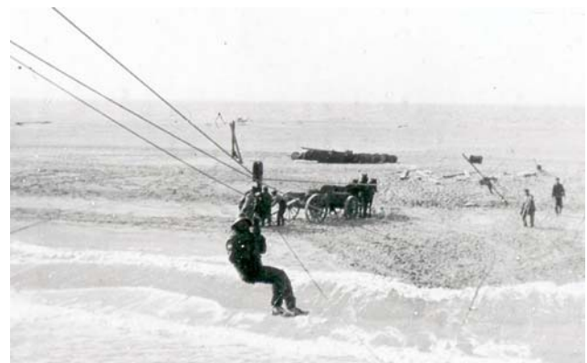
The breeches buoy in action, disembarking some of the crew of the barque Crofton Hall. The arrangement was later used to salvage food and parts of the ship such as the sails
