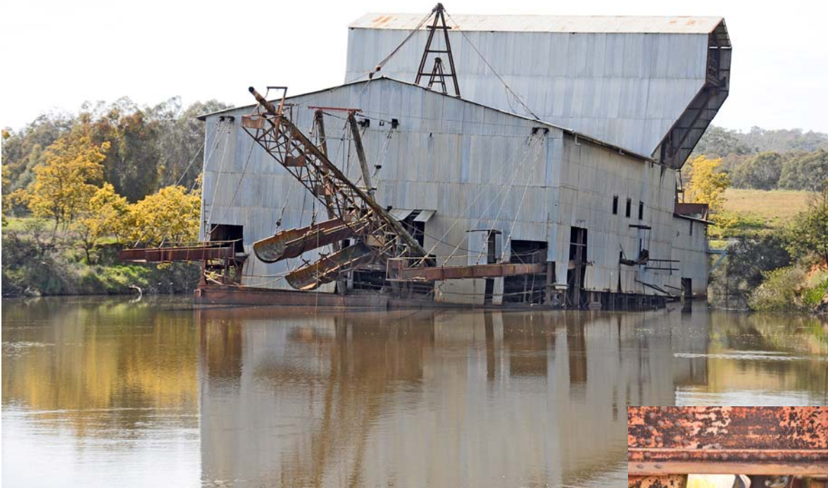
A stern view (above) of the massive, derelict dredge on Reedy Creek at Eldorado in Victoria. The spoil is ejected out along the chutes.
