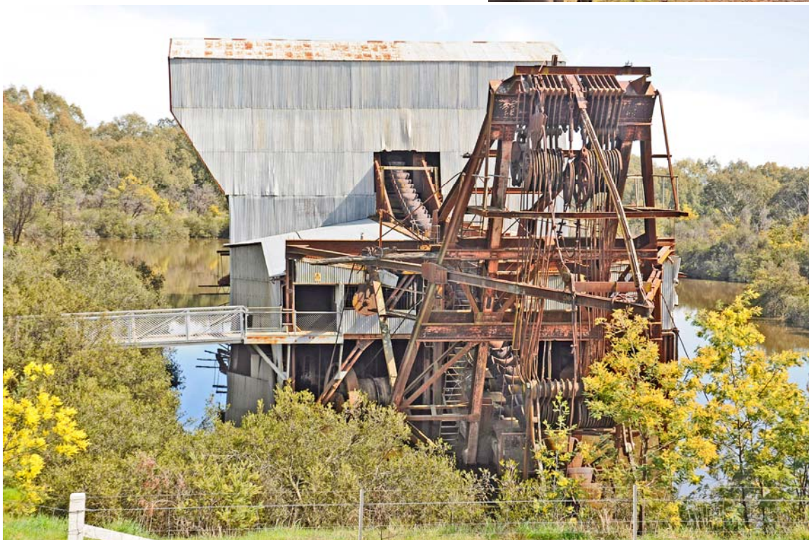
A view of the control room (above) and the bow (left) of the dredge showing the gear necessary to raise and lower the bucket ladder
