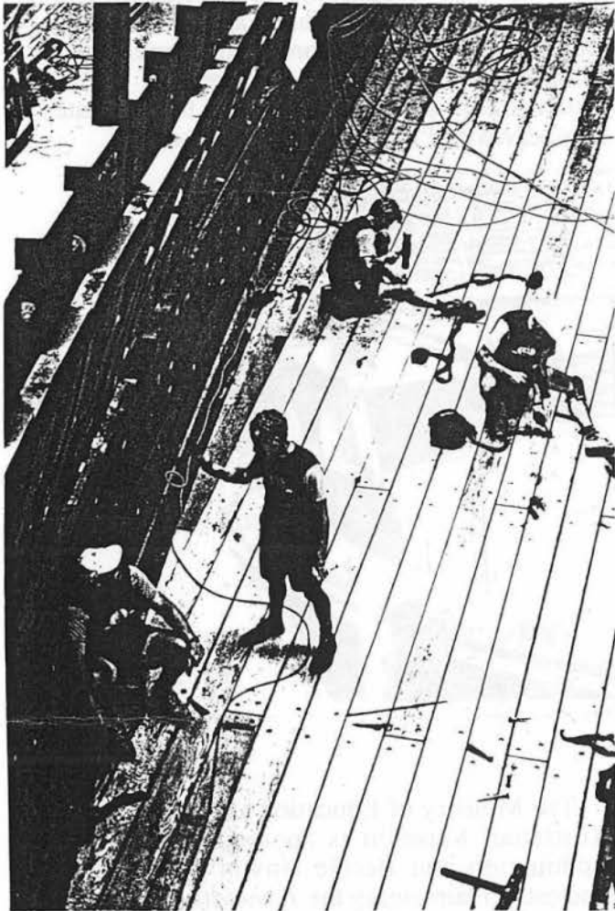
Photo: J. Lancaster. Caulking the lower deck.
