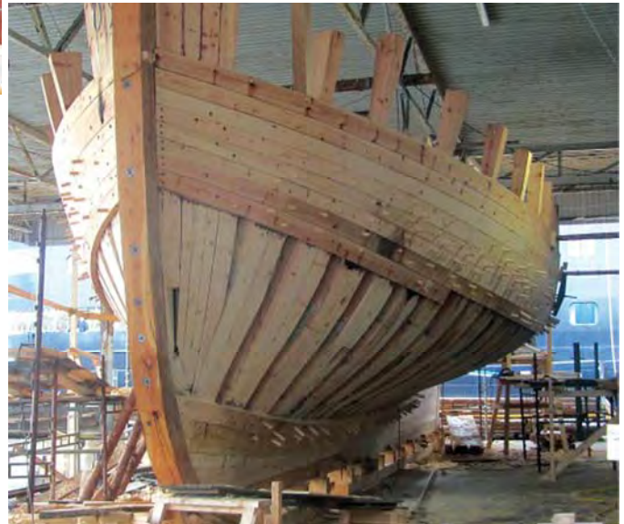
The bankskoyta under construction
